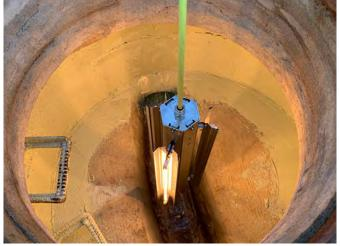
Der **Schachtheizer** (manhole heater) is a mobile, electrically operated device for heating manholes in the course of rehabilitation work with synthetic resins.
