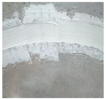
**Harz12** is a pasty Epoxy resin composed of two components for the rehabilitation of waste water systems with approval by DIBt.
