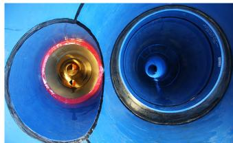
**Harz8** is a permanently flexible and fast curing Epoxy resin composed of two components for the manual application. Harz is approved by the DIBt for liner connections to manholes and the sealing of annular gaps on PE.
