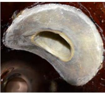
**SIDELINER**<sup>TM</sup> is a two-component Epoxy resin system for impregnating needle felt hats used for the robotic repair of lateral connections.
