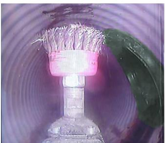
**SIDELINER**<sup>TM</sup> is a two-component thixotropic Epoxy resin system for impregnating needle felt hats used for the robotic repair of lateral connections.
